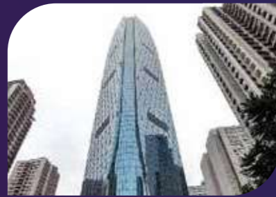
One Island East Taikoo Place, Quarry Bay
