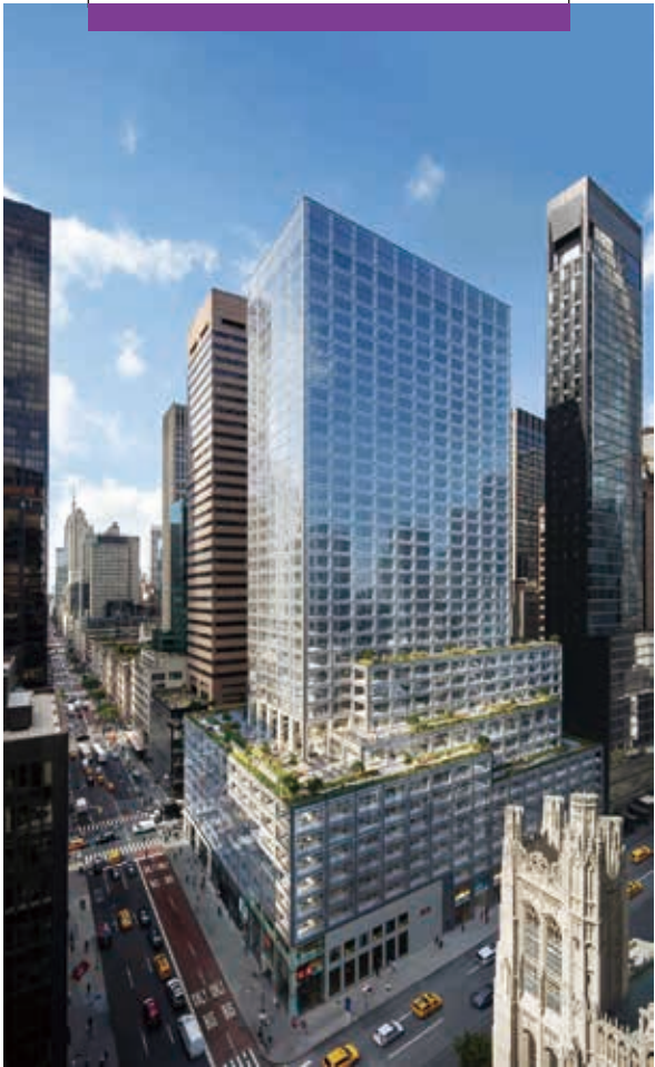
660 Fifth Avenue, New York City, USA This 41-storey office tower in Midtown Manhattan was built in the 1950s and renovated in the 2020s. As part of the renovation the passenger and service lifts were modernised and a destination-based dispatch system was installed.
