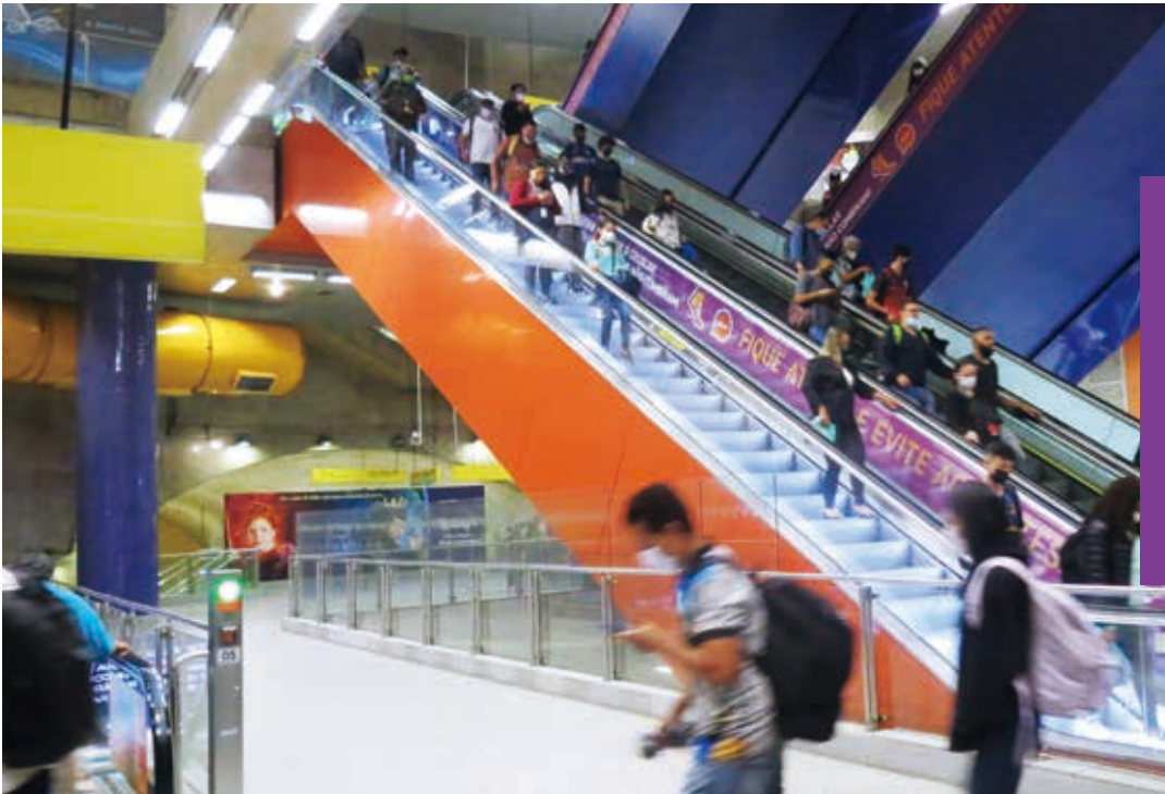
Pinheiros and Faria Lima stations, São Paulo, Brazil Pinheiros and Faria Lima are metro stations on Line 4-Yellow of the Brazilian São Paulo Metro, operated by ViaQuatro. Anlev has delivered several heavy-duty escalators and a lift to these stations.
