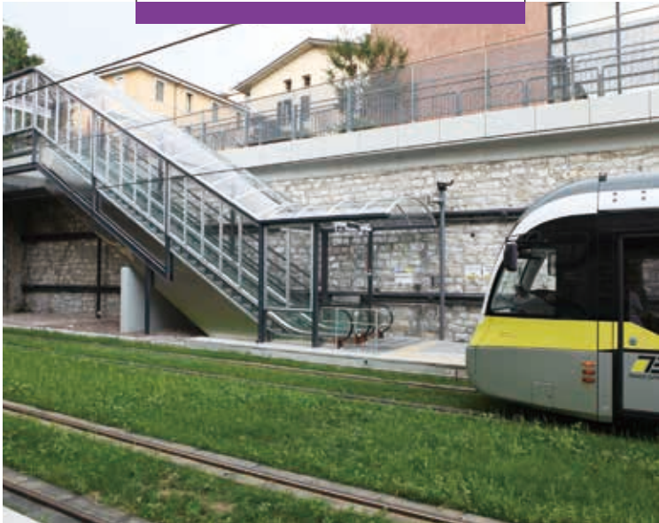
TEB Borgo Palazzo, Bergamo, Italy Anlev has supplied escalators to the Borgo Palazzo railway station in the city of Bergamo, Italy.
