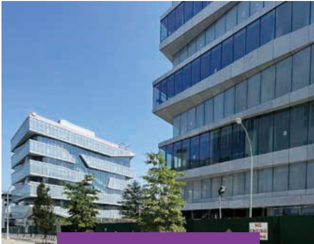
Columbia University, Manhattanville Campus, New York City, USA Columbia University is a private Ivy League research university and the oldest institution of higher education in New York. A large number of elevators have been installed.
