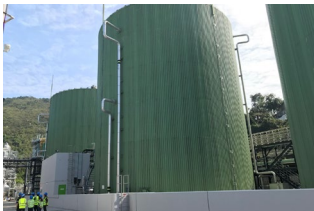
Anaerobic digestion tank 厌氧消化罐
