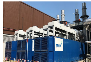
Combined heat and power (CHP) generator 热电联产发电机
