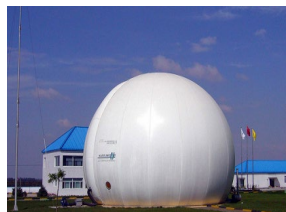
Biogas storage tank 沼气储存罐
