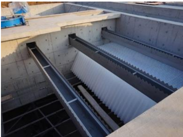
Lamellar of AMSFS II under installation 安装在磁介质高效沉淀池的斜管
