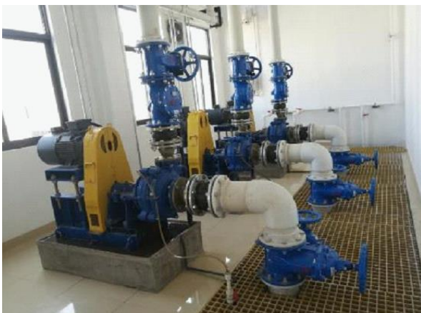
Sludge Pumps of AMSFS II 磁介质高效沉淀池的污泥泵
