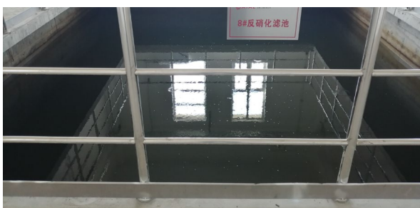
ASDBDF under operation 运行中的ASDBDF
