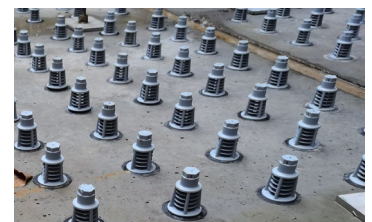
Water and air distribution system in Filter Tank 滤池配水配气系统
