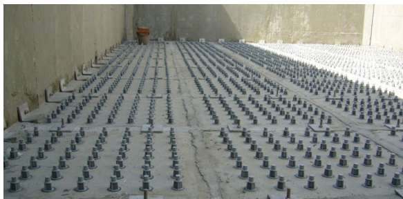
Water and air distribution system of ABAF 曝气生物滤池的配水配气系统
