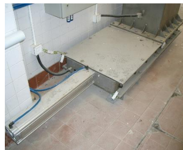
Air Intake Valve and Discharge Valve 入口阀及出口阀
