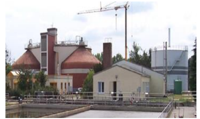
Bamberg Sewage Treatment Plant in Germany 德国班堡污水厂
