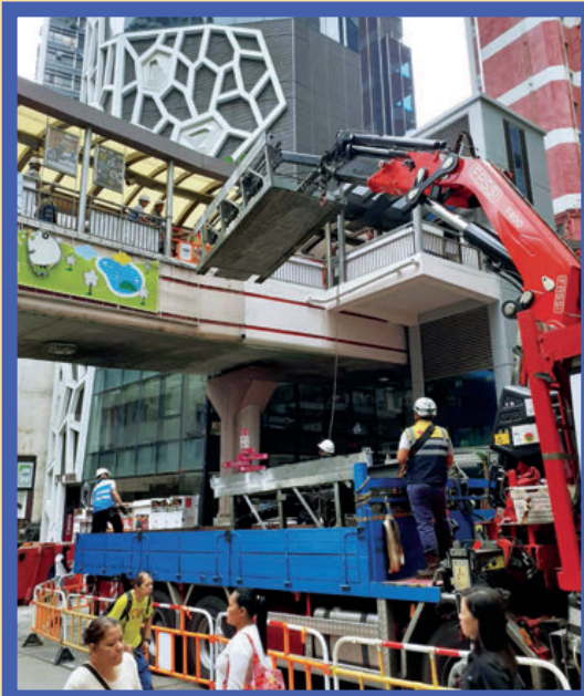
Conducting hoisting in busy, narrow streets within a very short time means that meticulous planning is required in advance. Hoisting was only allowed on Mondays to Fridays at 10-11 a.m. and 2-3 p.m. to minimize road traffic disruption.
