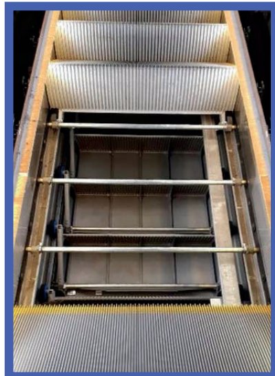
Footsteps were customized and used for worker safety and will be reused at other sites.
