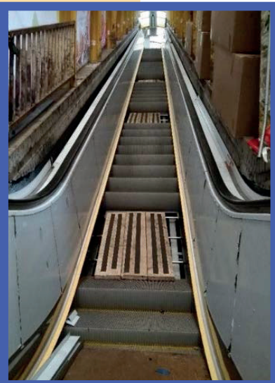
Footsteps were customized and used for worker safety and will be reused at other sites.
