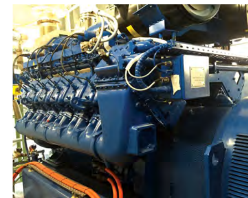
Combined Heat and Power Plant (CHP) 熱電聯供系統
